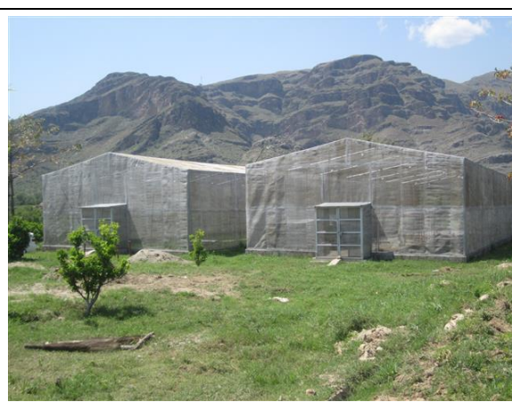
Figure 13: Commercial screenhouses at Sherkhana, KP built with assistance from ASF Pakistan.
